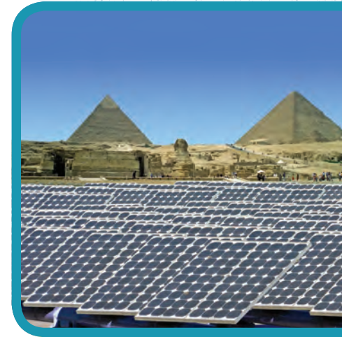
Egypt is using solar panels to improve its electricity system.
